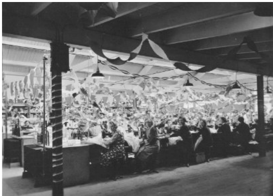
Tower 2 Works decorated for the coronation of King George VI.
